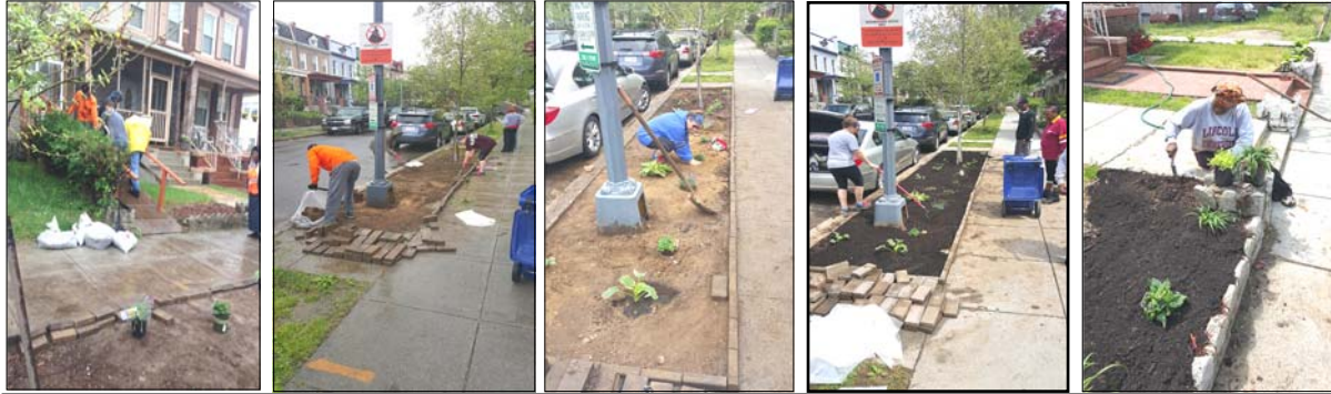
Franklin Street neighbors dig in, up, out, and plant!
